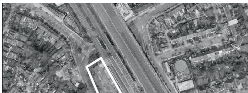
Figure 1: The Bunns Lane Car Park Development Site
